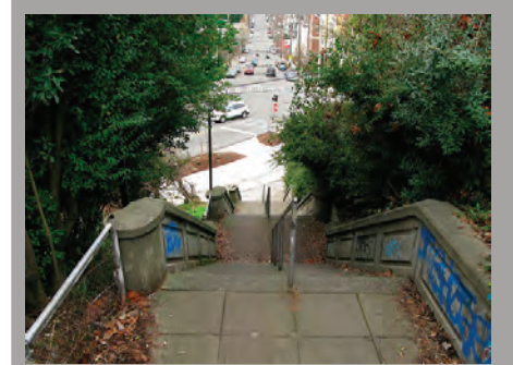
Galer staircase to Queen Anne Avenue - Courtesy of Rob Ketcherside
