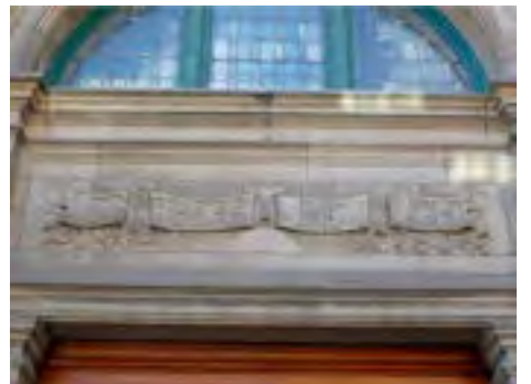
Figure 2: Entablature over the door of the Edinburgh, Scotland Carnegie Library
